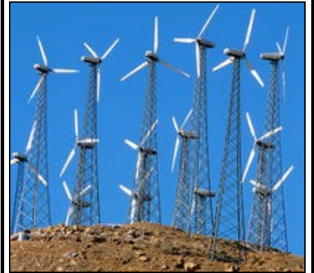
Fig 8(b) Lattice tower
